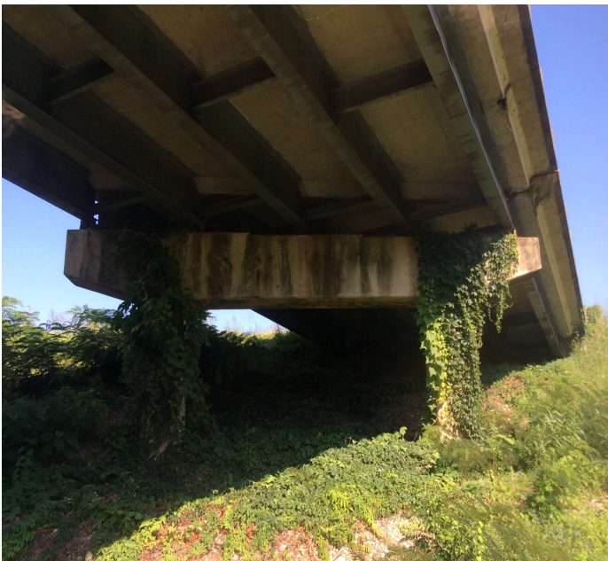
PHOTO 1 Description Bent 2 vines growing on columns & cap.
