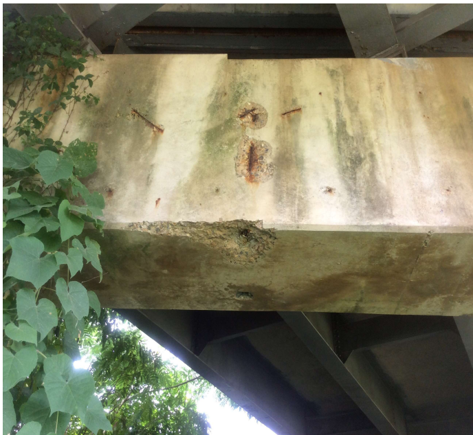
PHOTO 1 Description Caps at bents 2 and 3 have large spalls with rebar exposed
