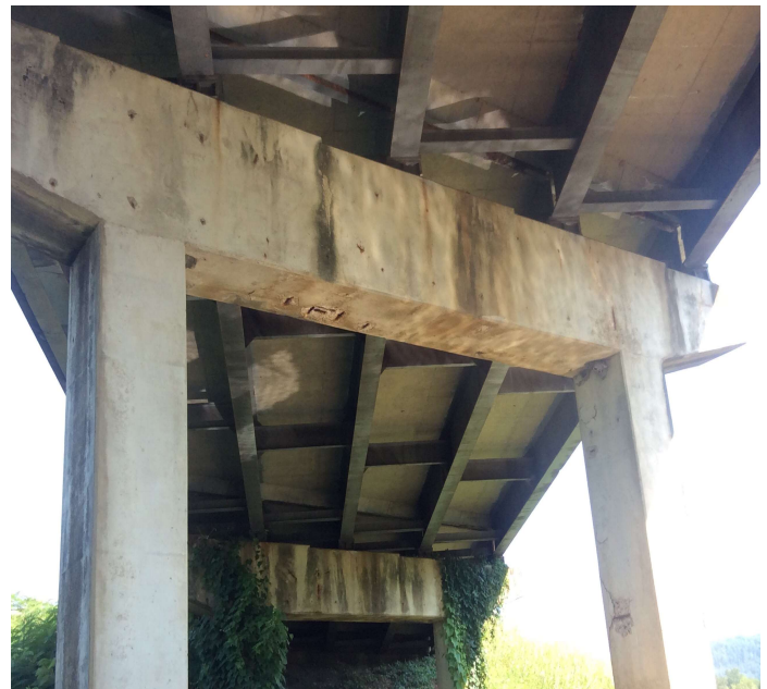
PHOTO 2 Description Bent 3 looking back, spalls with exposed rebar on columns & cap.
